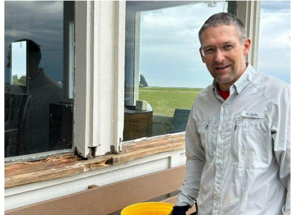
*Todd Hahn works on removing the dry rot on the front window sills.*
